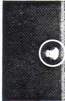
Figure 3A. Hex cap bolt holding top to bottom
